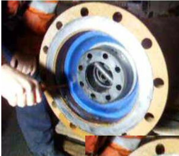
Screwdriver is forced between the 12" seal and the 10" pipe wall
